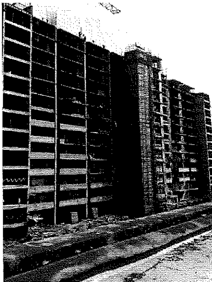
Side view of Block-C
