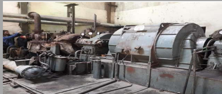
A photograph of steam turbine with generator installed for power generation at KSCML,
